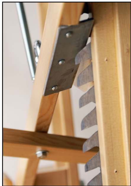
Ratchet and underside of draw down lever.
